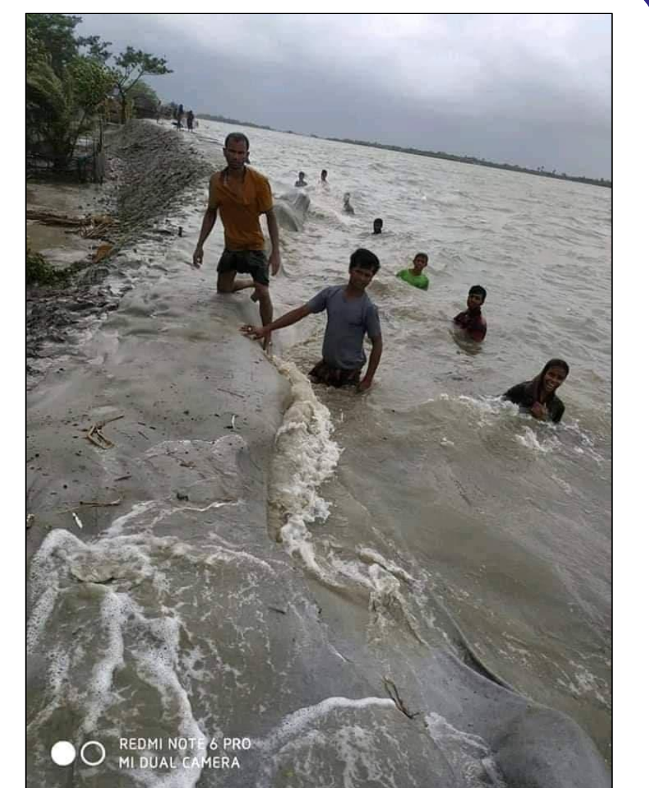
Fig 4: Community effort to repair a coastal dike before cyclone Amphan landfall.
