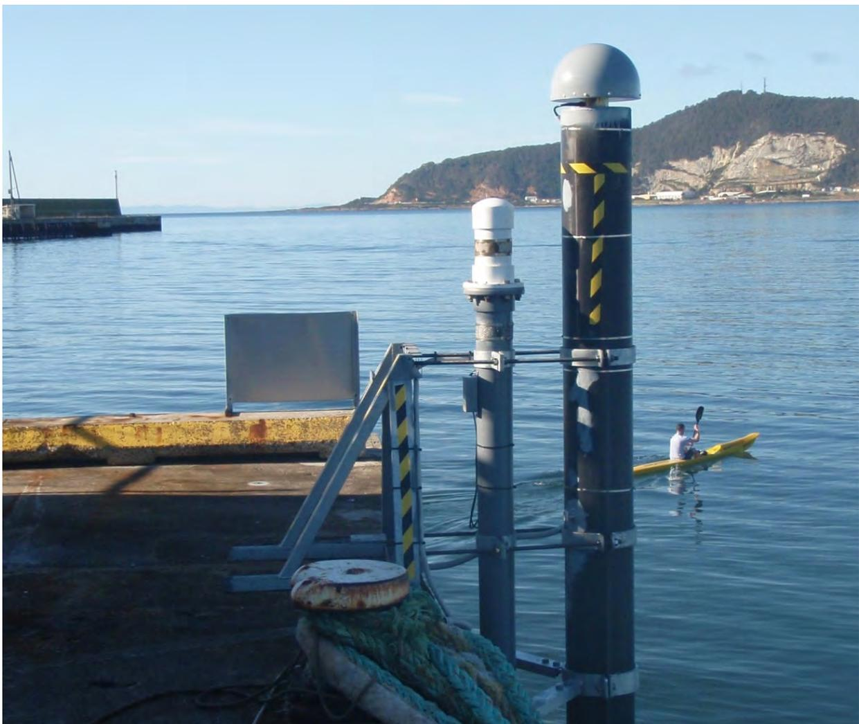
**Figure 6.4** An acoustic tide gauge at Burnie in northern Tasmania, Australia, and, to its right, a special pillar with a GNSS antenna on top. Photograph courtesy of Geoscience Australia. From Pugh and Woodworth (2014).
