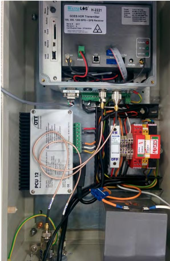
**Figure 7.7** The inside of a tide gauge electronics cabinet. A Waterlog GOES HDR transmitter is shown at the top of the cabinet while the lower part contains a power supply and back up battery. The data logger is located behind the HDR. (Photograph NOC).
