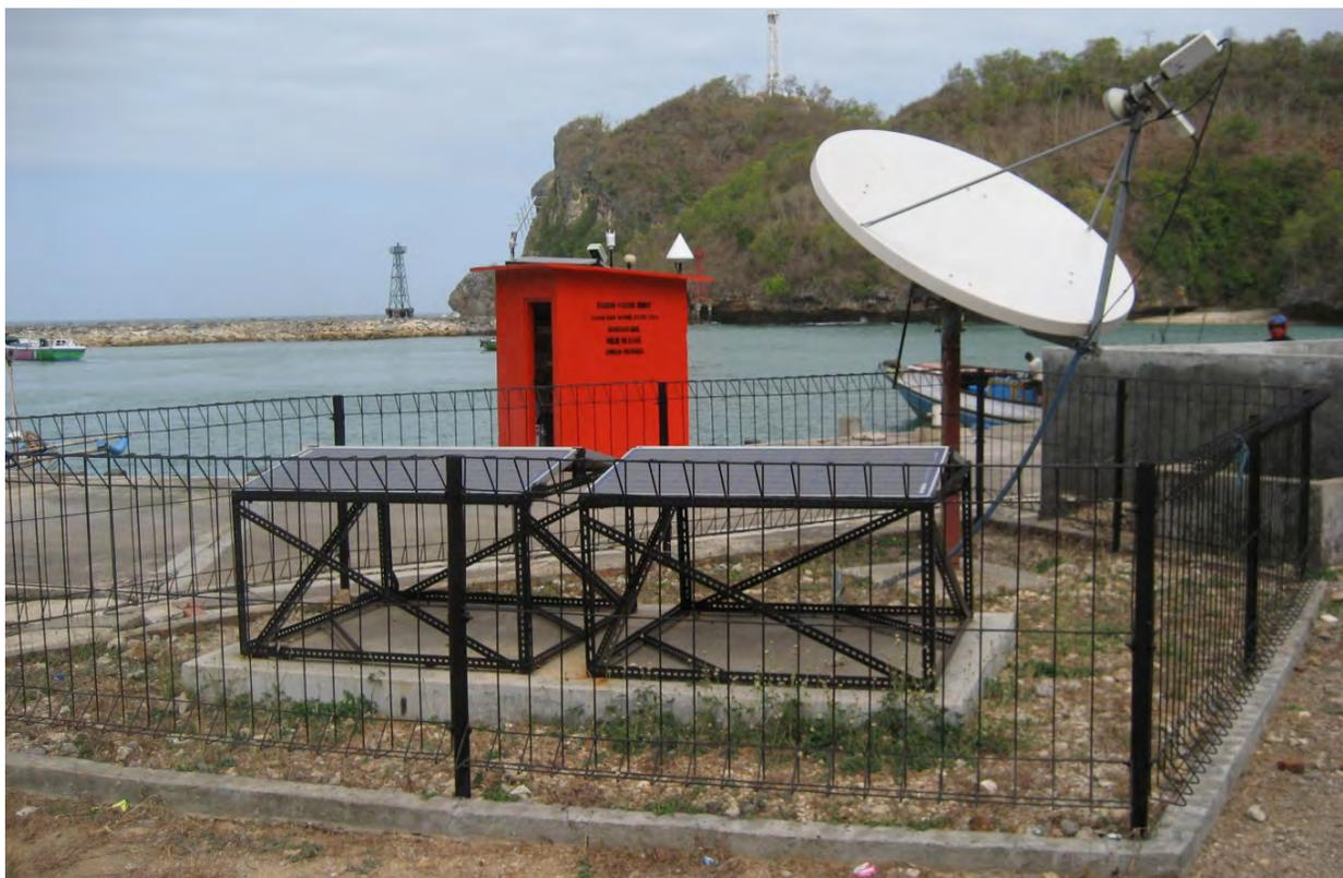
**Figure 7.5** A VSAT dish alongside a tide gauge in Indonesia. This station is also equipped with an OTT Kalesto radar gauge and GPS receiver. (Photograph Tilo Schöne, GFZ).
