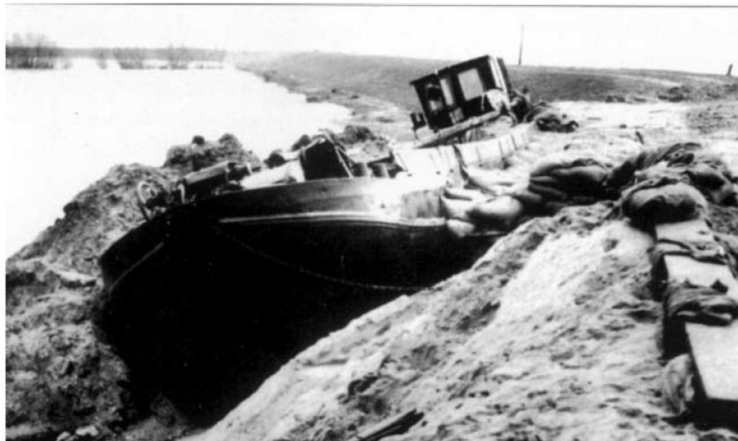
Figure 9. The ship that closed the dyke breach and saved the central parts of Holland from flooding
